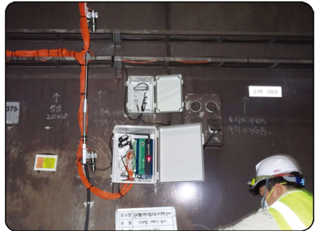
[ADL-16V Installation in tunnel]
